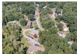
Apple Ridge Condos Maynard Roofing • 90 Units, 15 buildings
