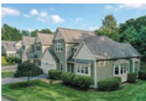
Deerfield Estates Hopkinton Painting 48 town houses
