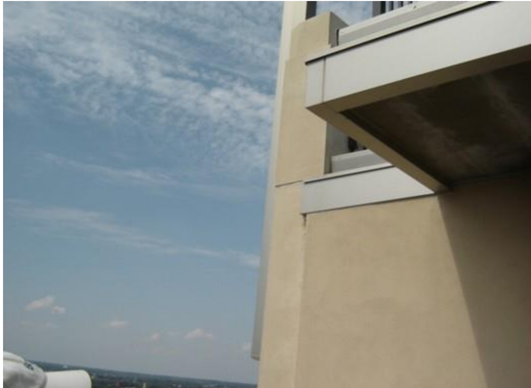
View of underside of metal flashing and balcony from terrace
